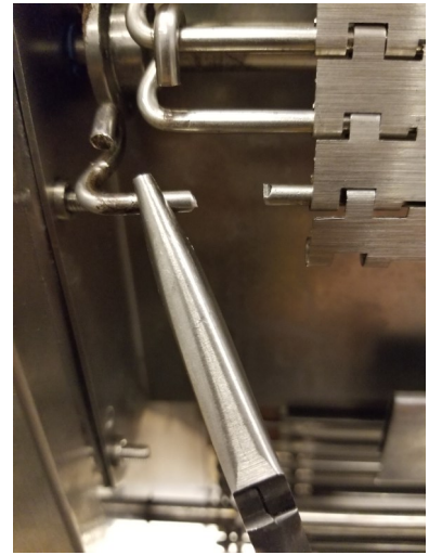
View of the cut wire
