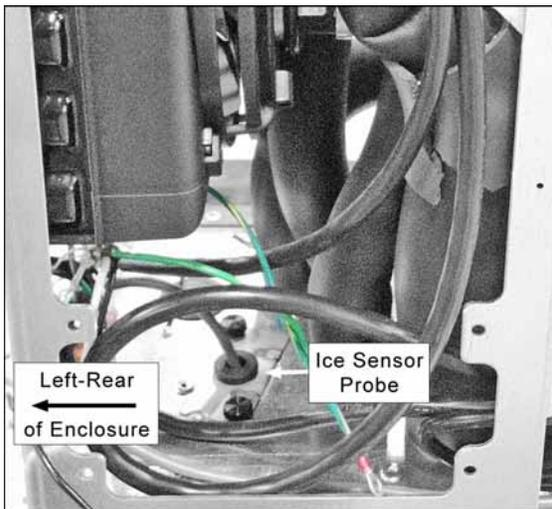
Figure 6-12 - Ice Sensor & Control Module Locations
