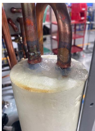
Joint between copper and factory foam is sealed with RTV.
