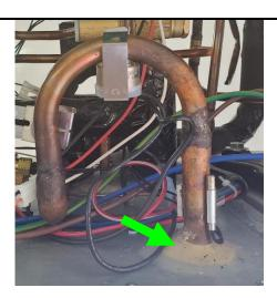
Using RTV, place enough over permugum to create a seal on the inlet and outlet of the evaporator.
